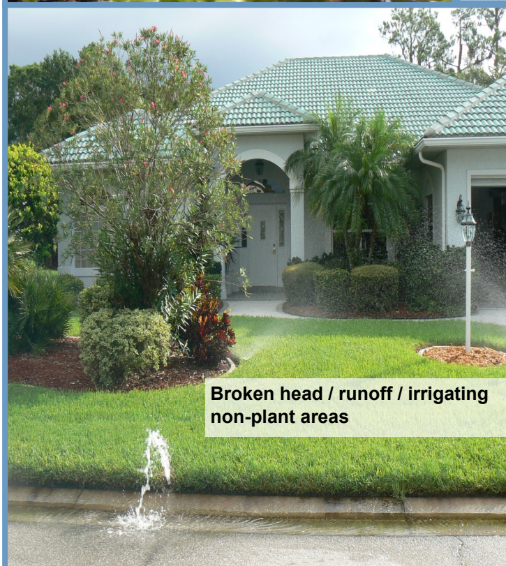
Poor design; irrigating non-plant areas
