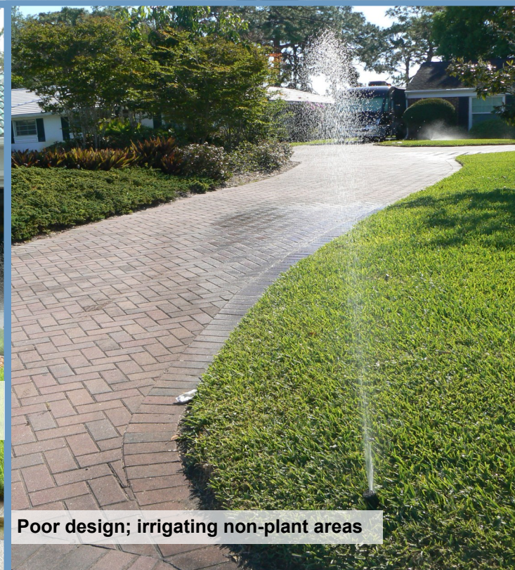
Broken head / runoff / irrigating non-plant areas
