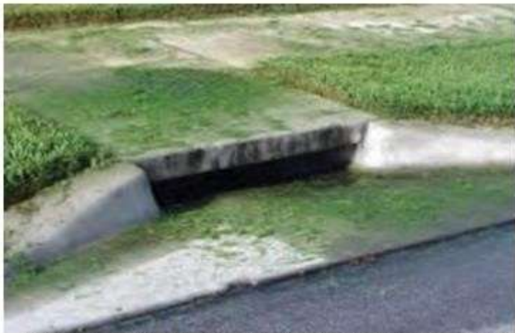
Remove clippings from impervious surfaces. These nutrients are going straight to a water body. Photo courtesy of FDEP
