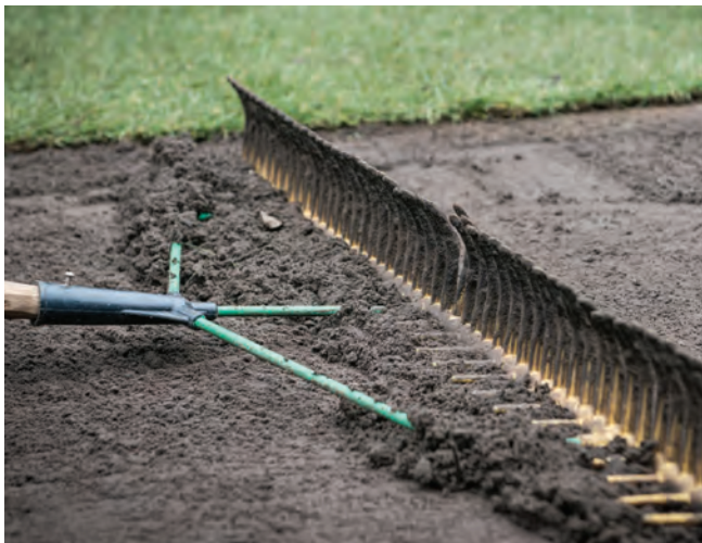
Figure 14-4. Final hand raking in preparation for sod laying.
