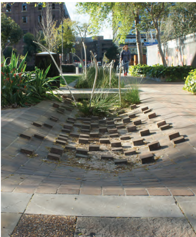
Figure 10-22. Bricked lined swale in an urban setting for drainage. Additional brick and plants are placed to slow water flow.
