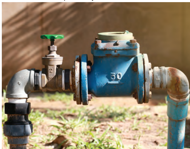
Figure 10-6. Backflow prevention device (check valve).
