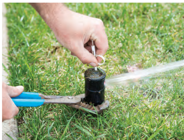
Figure 10-25. Adjusting sprinkler heads to avoid overspray.
